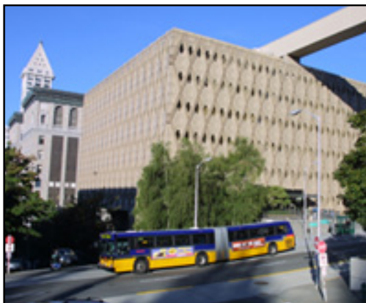
The new system took into account not only County administrative buildings but also fleet management facilities.
